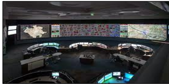
Main Operational Room
